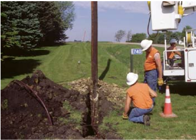
(From left) Slaichert, Clevenger and Weiskamp position a new primary underground electrical cable under an existing telephone line, because the underground electrical cable needs to run deeper than the telephone wire.
