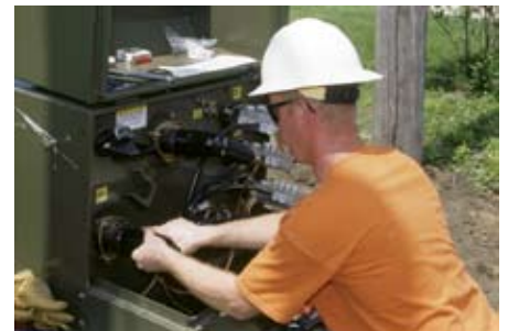
Anderson double-checks his work as he prepares to energize the electrical connection in the transformer. The unit converts the 7,200 volts from the underground cable to 110 and 240 volts for the co-op member's use.
