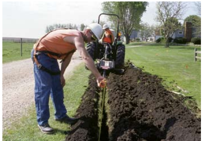
Back on the ground, Grove operates the trenching machine as Weiskamp checks the trench’s depth. The next step is laying the cable into the trench and covering it with a 12-inch layer of fill dirt.
