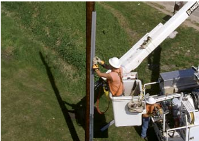
Weiskamp nails a plastic shield (called a “U-Guard”) over the electric cable attached to the riser pole to protect the cable from wear and to prevent anyone from coming into contact with the underground cable.
