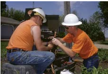
Clevenger (left) and Anderson install an elbow to the end of the underground electrical cable and attach it to the transformer. They also connected the secondary household voltage wires that go to the pole.
