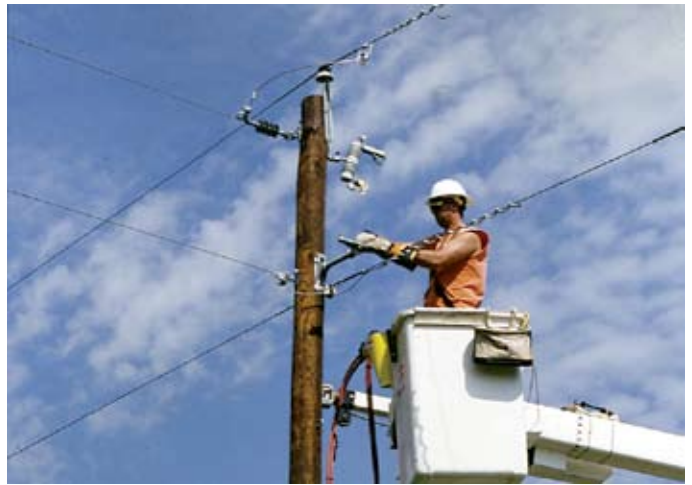
Weiskamp installs a lightning arrester on a pole bracket. The next step in the process is hanging the underground electrical primary cable on the riser pole, next to the lightning arrester.
