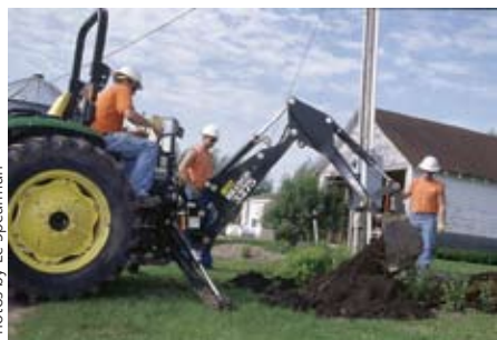
(From left) Brent Grove, Andy Weiskamp and Tim Slaichert use a backhoe and hand shovels to expose existing utility connections at the pole that connect to the homeowner's electrical service.
