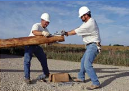
3 Matt Weiland, field service foreman (left), and Steve Ralston, field service rep, "framed" the new pole by attaching new insulators and hardware.
