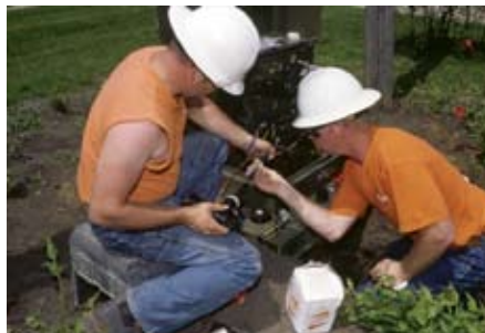
To protect the electric cooperative's transformer case and internal windings from voltage surges caused by things such as lightning, Clevenger (left) and Anderson install an elbow arrester.
