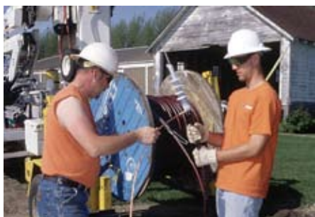
Clevenger and Buns twist exposed copper wires from the underground cable to create a neutral connection to a grounding rod, which will safely discharge excess electrical energy into the ground.
