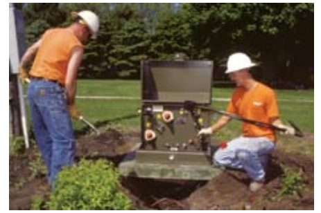
Clevenger (left) and Anderson pull the underground cable through the pad and place an elbow on the end of the cable, to create a safe connection when the cable is attached to the transformer.
