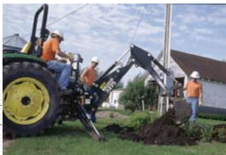
(From left) Brent Grove, Andy Weiskamp and Tim Slaichert use a backhoe and hand shovels to expose existing utility connections at the pole that connect to the homeowner's electrical service.
