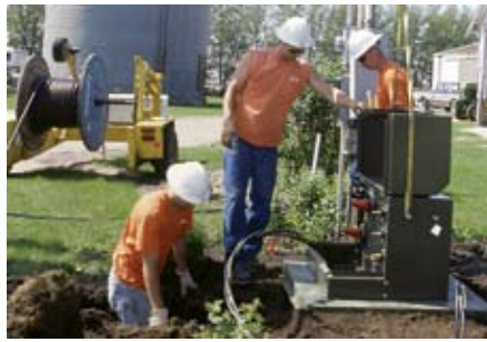
(From left) Buns, Weiskamp and Adam Anderson position the new electrical transformer on a base called a "pad." All of the electrical connections for the property owner's service will be made within this unit.
